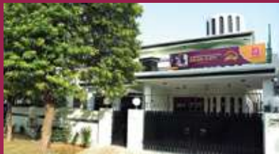
HOUSE NO# 141 V BLOCK, PHASE 5, DHA, LAHORE
